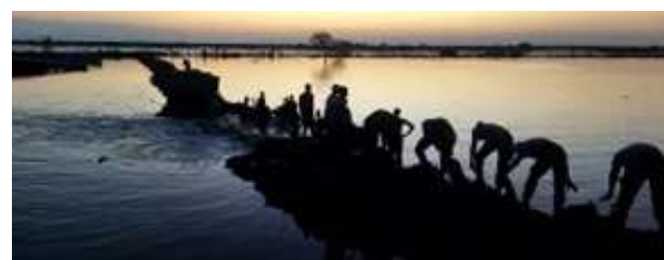
Pak METF human chain reinforcing breached section manually
