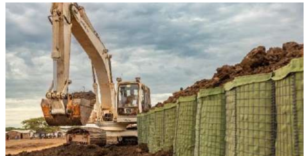
Pak METF excavator reinforcing HESCOs to enhance the protection of the IDP camp
