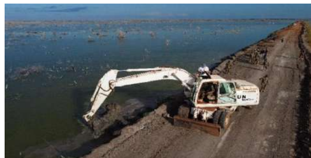
Pak METF-5 excavator reinforcing dyke astride only road of Bentiu – Main Supply Route
